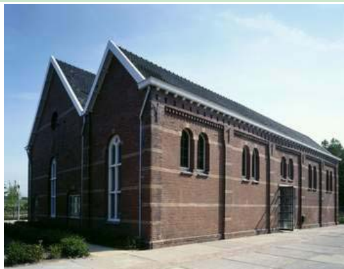
Machine building at Westergasfabriek, the venue for the conference (Photo: S. Swart)
