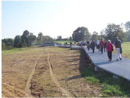
Image 4: Foreland bridge with river bridge in background
