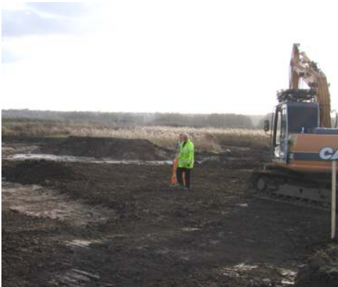
Construction of a new path on Crossness Southern Marsh
