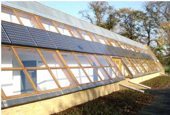
Exterior of the football centre, showing photovoltaic cells (photo: Studio E Architects)
